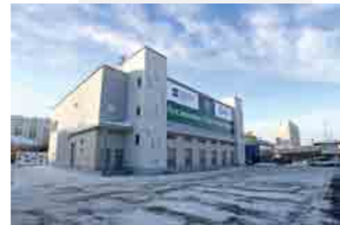
A new substation (90th anniversary of GOELRO plan) was commissioned into operation.
